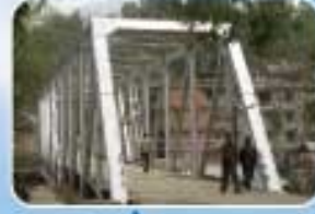
Hamilton Bridge Project BPO, Bhubaneswar
